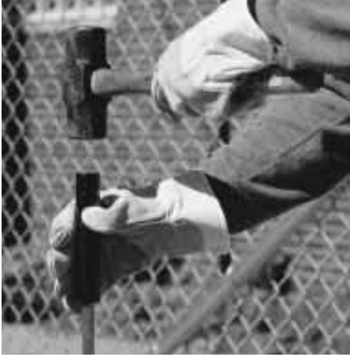
**ANSWER:** Use a driving sleeve or ERITECH® ground rod driver. If using a threaded rod, use the screw coupling and drive stud when driving the rod. For a plain rod, either steel or copper clad, use the CADWELD driving sleeve listed below.
