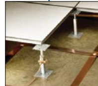
Signal Reference Grid (SRG)
