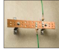
Telecommunications Ground Bar (TGB) and CADWELD Lugs
