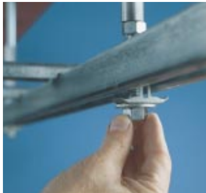
Mount strut to All-Thread Rod.
