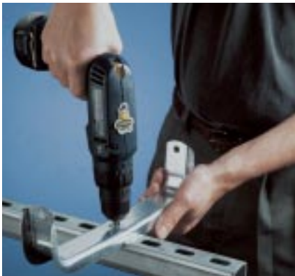
Mount U-Hook or Double J-Hook to strut.
