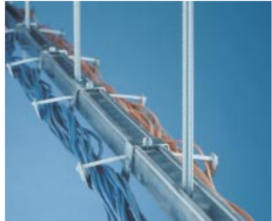
Double J-Hooks shown attached to standard strut
