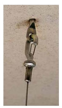
The Concrete Eyebolt Screw provides a simple and effective way to suspend electrical and mechanical devices from concrete and/or masonry structures. Requiring only a drilling machine capable of drilling concrete and a 5 mm diameter bit, the Concrete Eyebolt Screw eliminates the need for heavy, noisy and expensive equipment, such as powder actuated tools.
