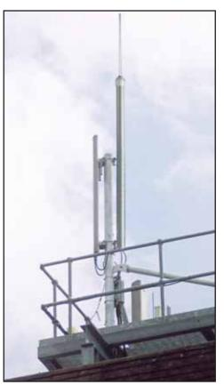
Illustrators representation of installed ERITECH Isolated Downconductor system
